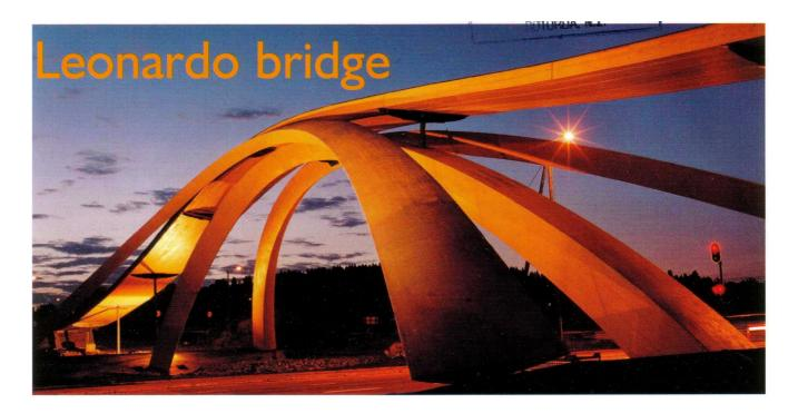
A bridge, originally designed by Leonardo da Vinci in 1502 has been constructed in Norway using modern glulam technology. The Leonardo bridge allows cyclists and pedestrians to cross the E 18 just outside the small town of As, south of Oslo.
