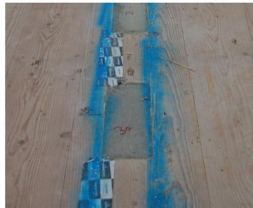
Figure 14: Notches in floor panels filled with concrete, from another job
