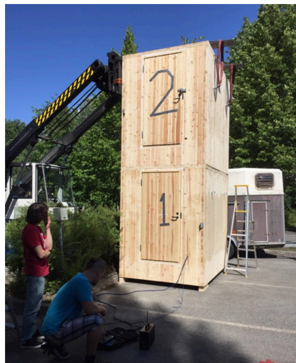
Figure 1: Sound insulation testing of CLT-modules at Karelia UAS premises. Image courtesy of Karelia UAS.
