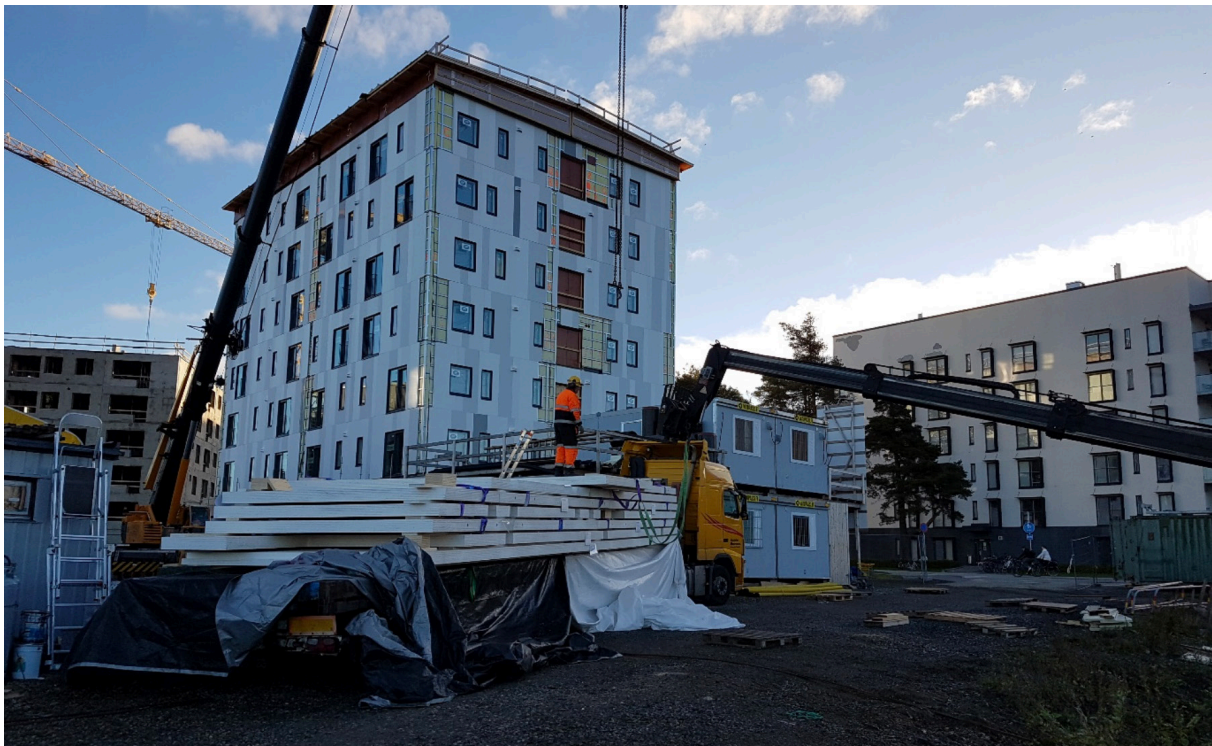
Figure 2: Construction crew at work unloading a truck at Lighthouse Joensuu site. Courtesy of Rakennustoimisto Reijonen.
