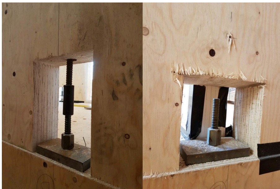
Figure 6: Restraining done from top of the wall with LVL-X wall installed afterwards. Courtesy of Rakennustoimisto Reijonen.
